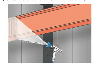
Alternatively, the steel can be coated by using a brush, roller or compressed air (PYRO-SAFE FLAMMOPLAST SP-A2 nozzle bore  $\geq 3.5 \, \text{mm}$ , PYRO-SAFE Dekorlack SP 2 top coat nozzle bore  $1.5 - 2.0 \, \text{mm}$ ).
